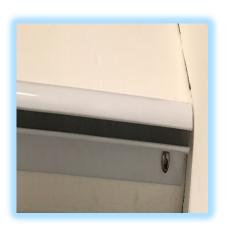
**Guide Description**: Track is mounted to the underside of support beam and screen fit inside the frames
