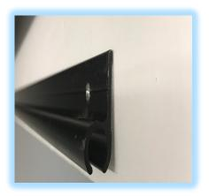
**Guide Description**: Track is mounted on the face of support beam
