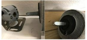
8. Insert the pivot pin into the roller idle end, ensure the rubber O-ring is in position to stop the pin sliding into the tube.
